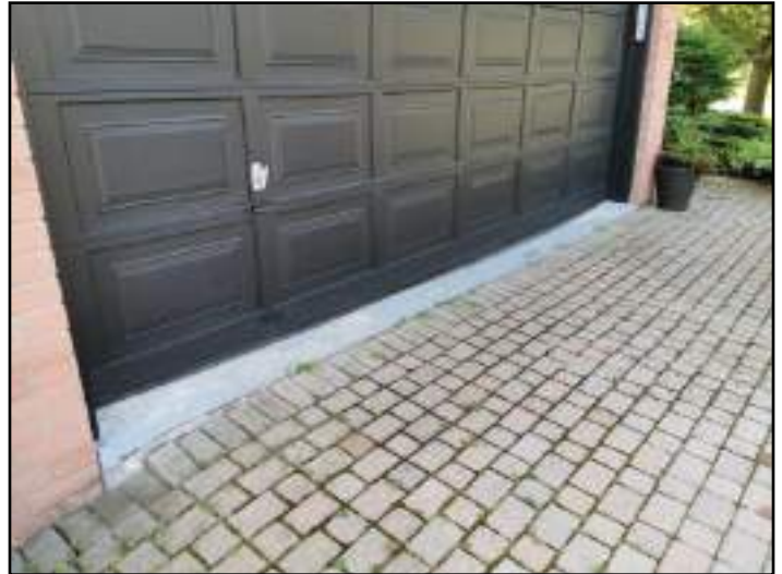
Improper slope
