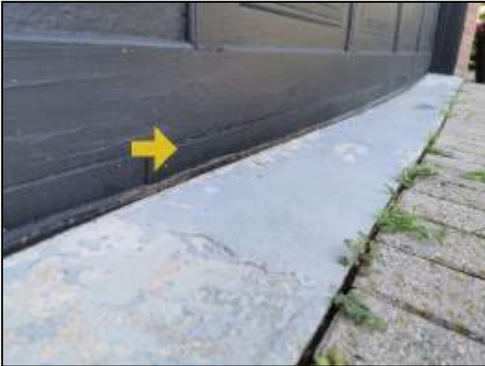
Improper slope
