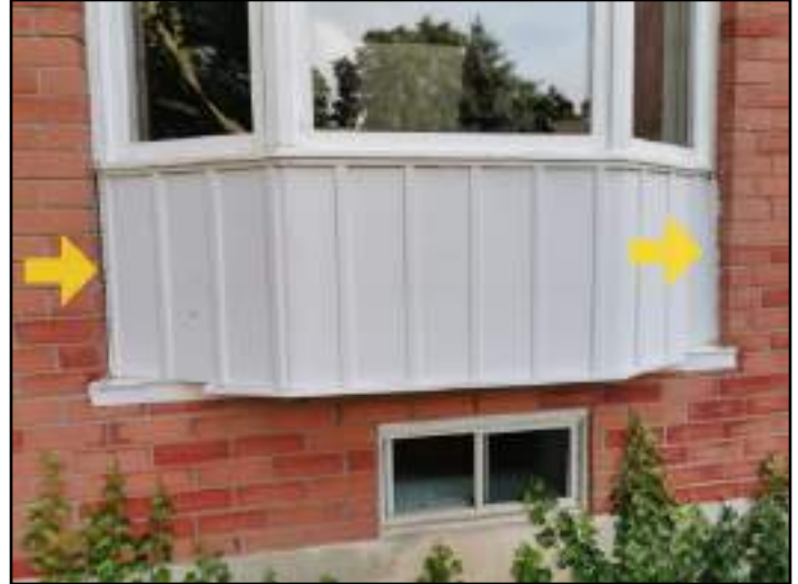
Caulking missing or ineffective
