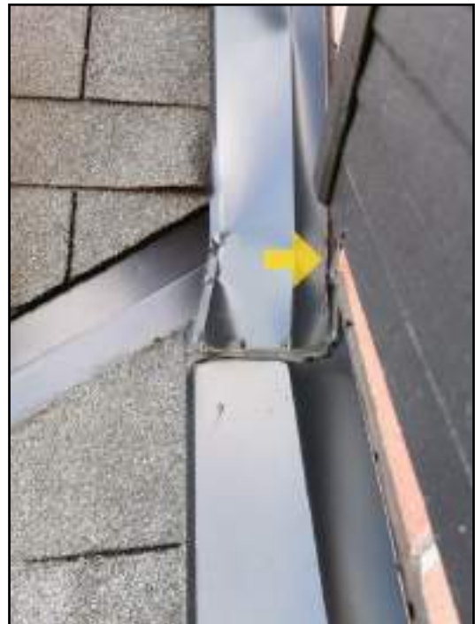
Replace old and cracked caulking.
