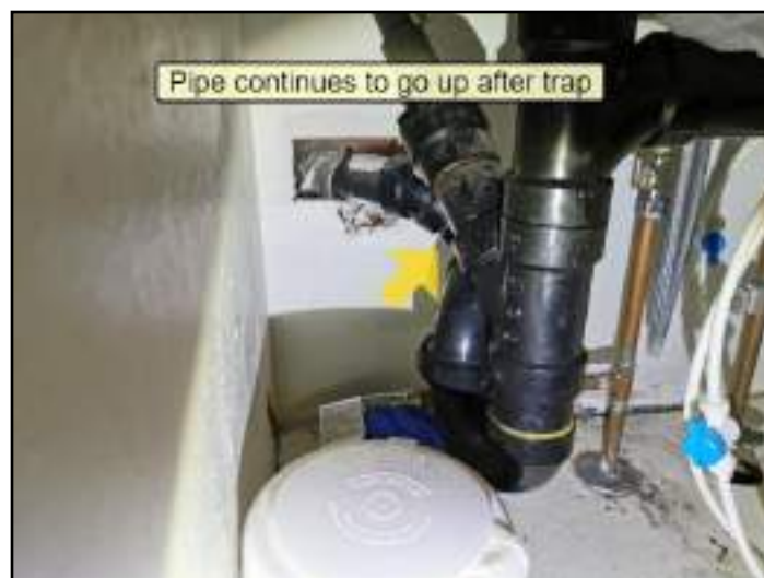
Poor manifolding of drain pipe
