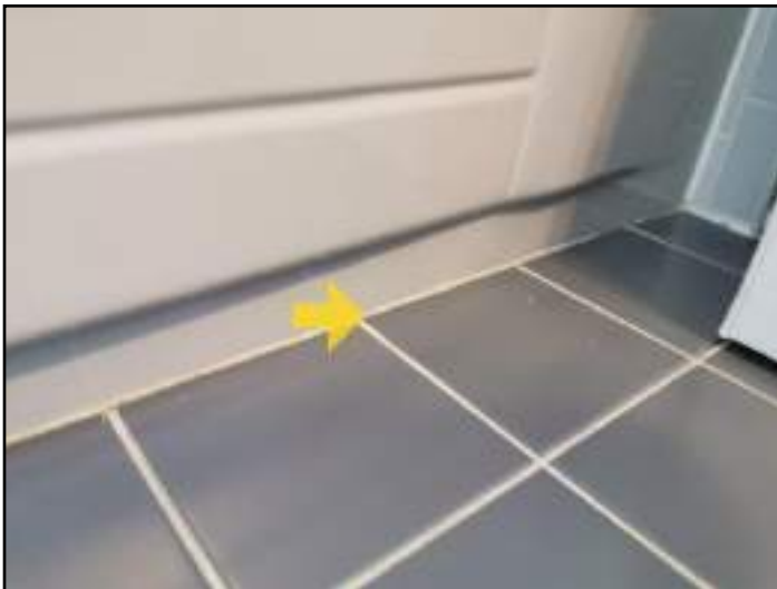
Caulking loose, missing or deteriorated
