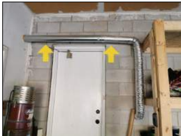
Not insulated in unconditioned space
