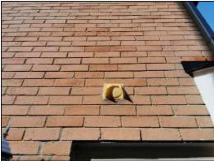
Cover damaged
