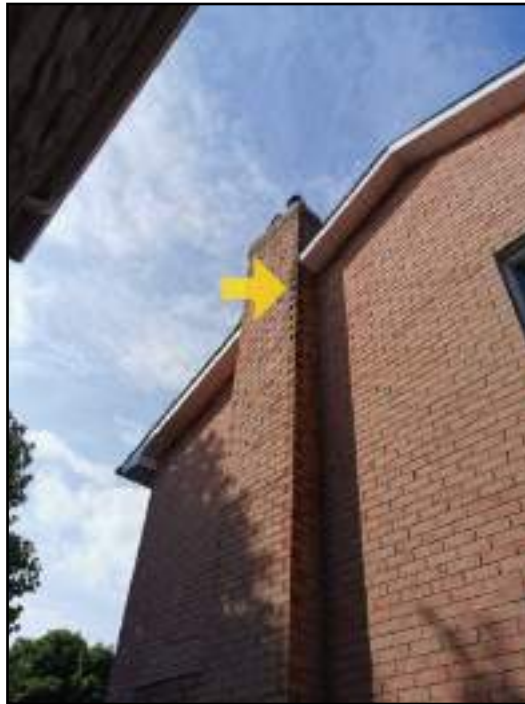
Loose, missing or deteriorated masonry
