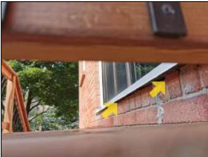
Caulking missing, deteriorated or loose
