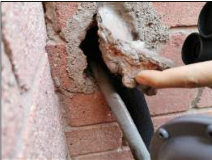
Poor seal at building
