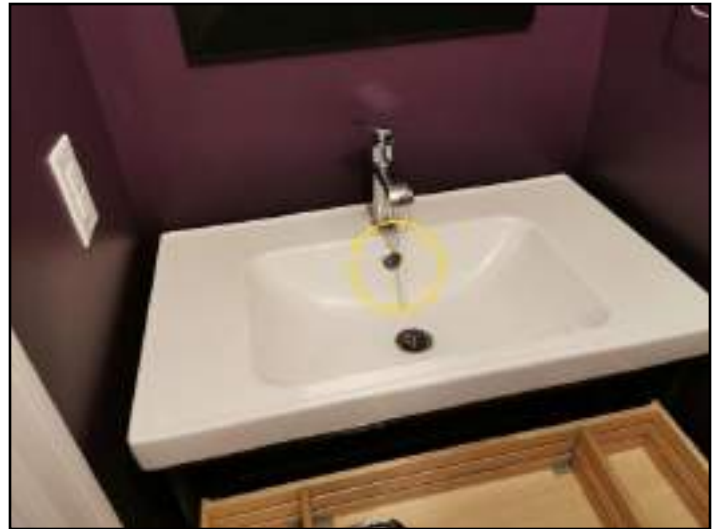
Overflows missing, leak, rust or...
