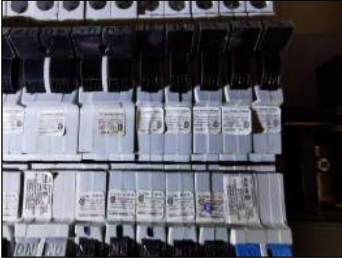
FPE (Federal Pioneer Electric) - Stablok...
