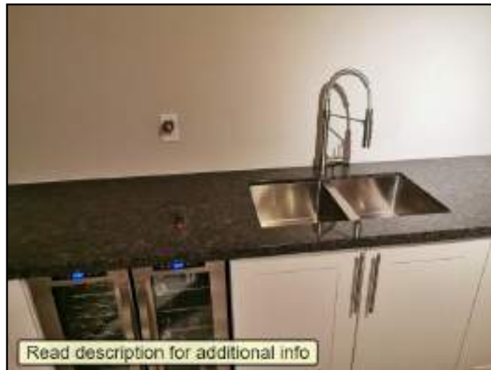
GFCI/GFI needed (Ground Fault Circuit...
