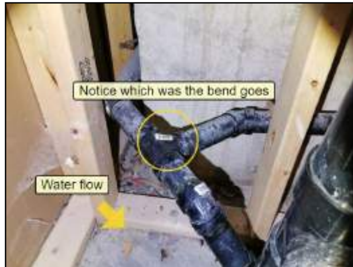
Poor manifolding of drain pipe
