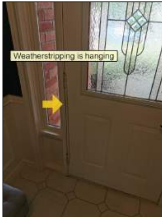
Weatherstripping missing or ineffective
