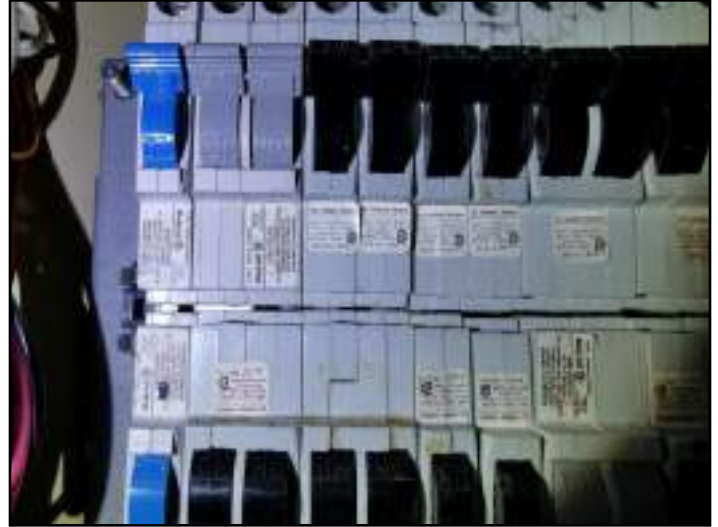
FPE (Federal Pioneer Electric) - Stablok...
