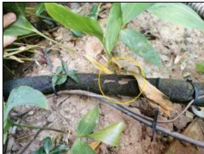
Insulation - missing
