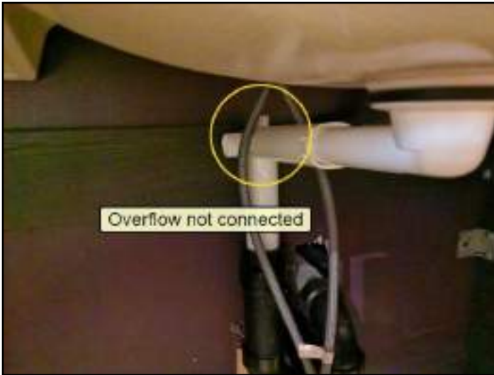
Overflows missing, leak, rust or...
