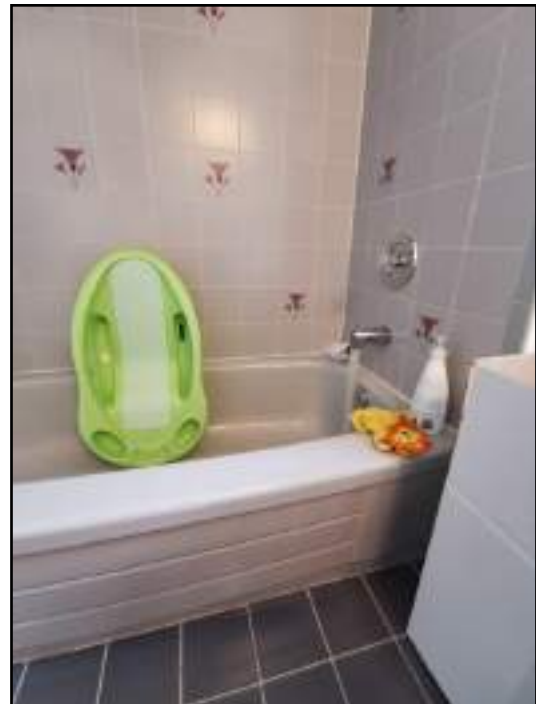
Caulking loose, missing or deteriorated
