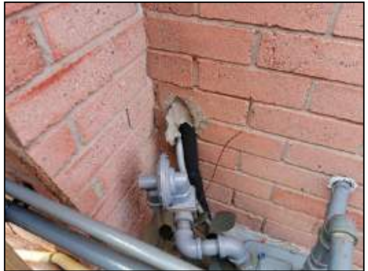
Poor seal at building
