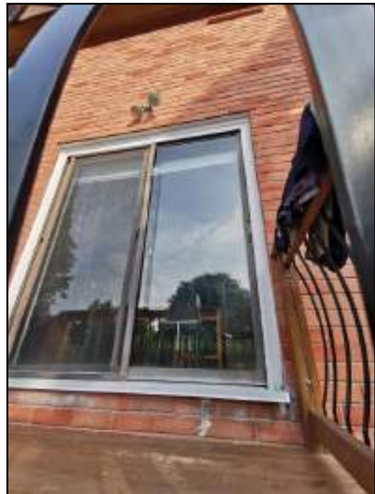
Caulking missing, deteriorated or loose
