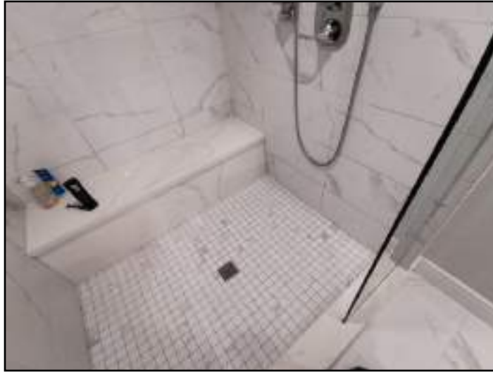
Caulking loose, missing or deteriorated
