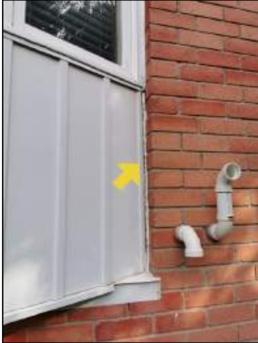
Caulking missing or ineffective
